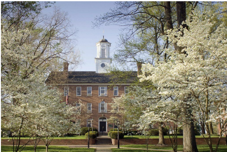
A shot of Brandon Hall, a very important building on campus.
