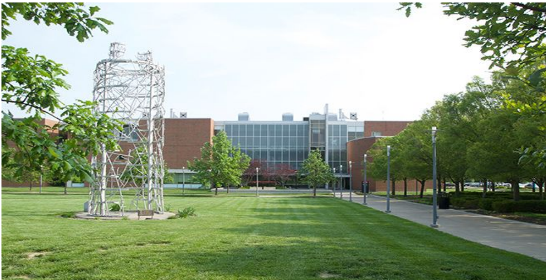
This is the path between two buildings and the sculpture is called the Quad.
