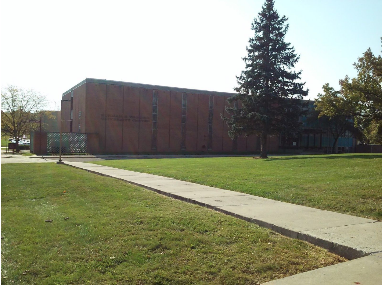
This is the Norman Ward University Center which is scheduled for demolition as they already have a building to replace it.
